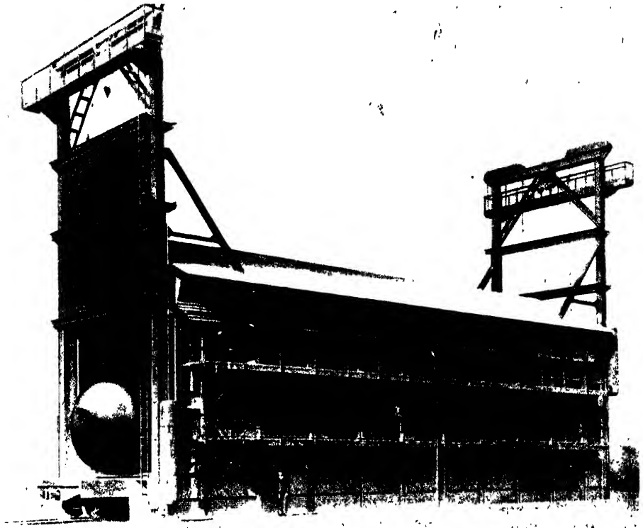
FIGURE 359. Large stress-relieving furnace, in the plant of the Sun Shipbuilding & Dry Dock Co., Chester, Pa. Used for stress-relieving welded pressure vessels and other welded structural work and for annealing large steel castings. Inside length is 80 ft and inside width 18 ft. (Courtesy Sun Shipbuilding & Dry Dock Co.)
